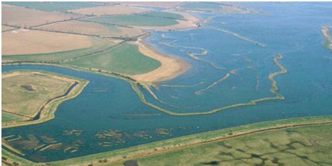
Aerial view of the Abbotts Hall managed realignment at high tide showing the flooded land behind the breached sea wall.
