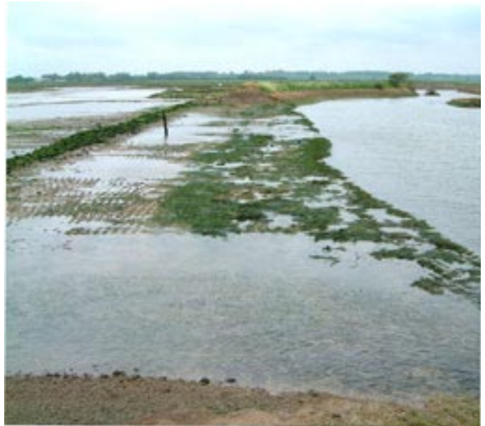
The sill at the main breach, designed to meet the oystermen's concerns
