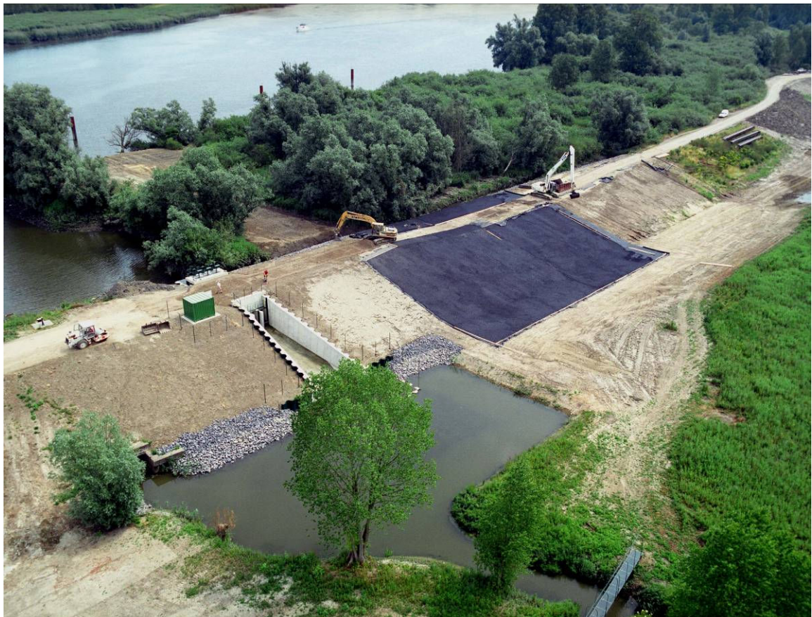
Figure 5 The inlet sluice and overflowing dike at Lippensbroek
