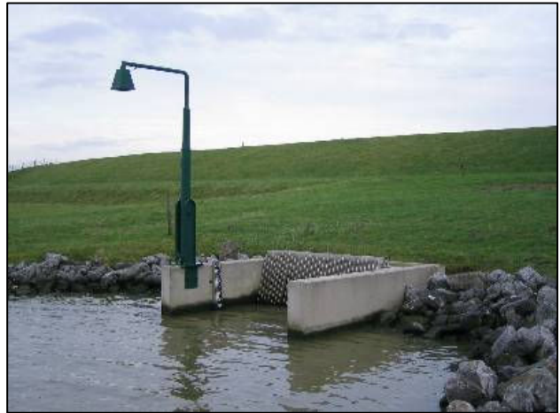
Landward side of culvert in primary dike
