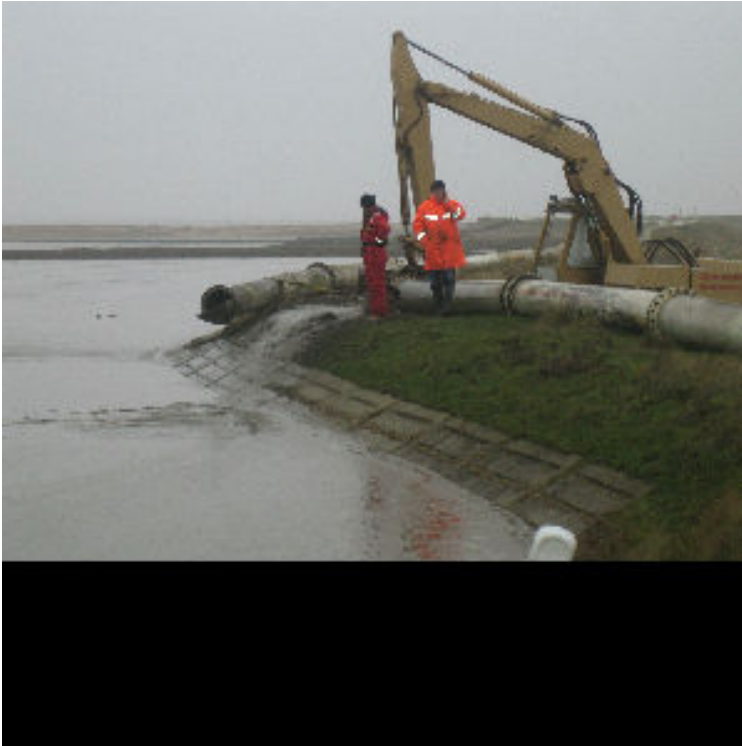
Pumping the dredged material onto the foreshore
