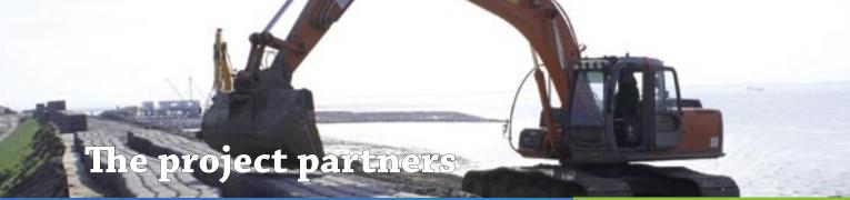
The seaward side of the new dike is strengthened with a layer of open asphalt. This layer is covered with soil allowing grass to grow on.
