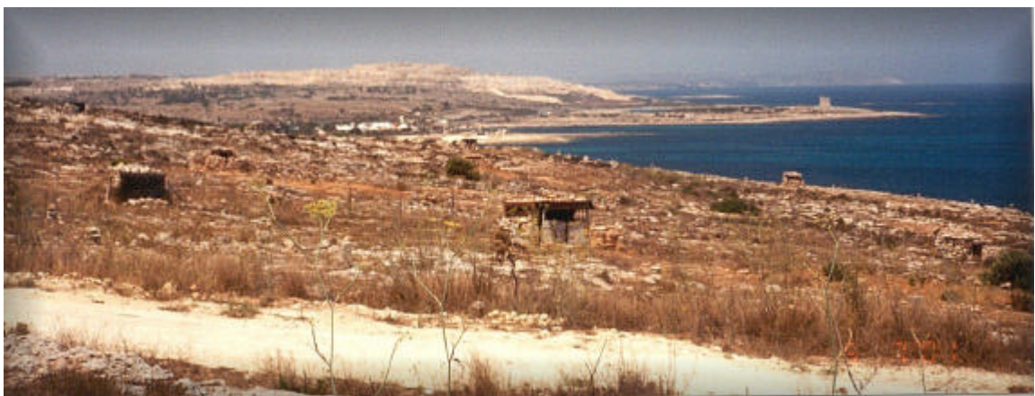
Photo 10: Maghtab - Landfills were placed on coastal locations to safeguard the underground water resources inland.
