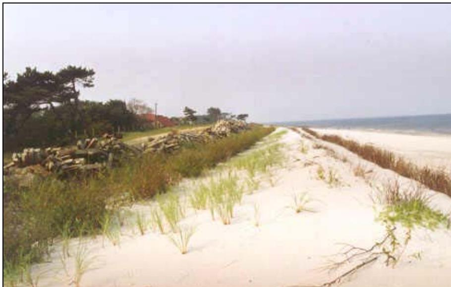
*Fig. 18: Concrete's sleepers seawall, Kuznica region, 1992 (photo by K.Furmanczyk).*
