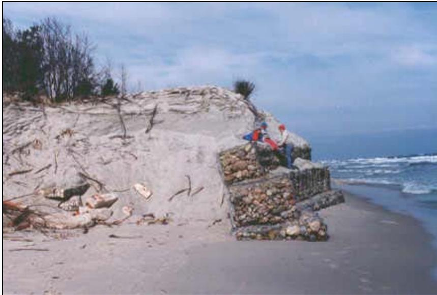
*Fig. 23: Seawall made with gabions lying over geotextil, Jurata, 1995 (photo by K.Furmanczyk)*
