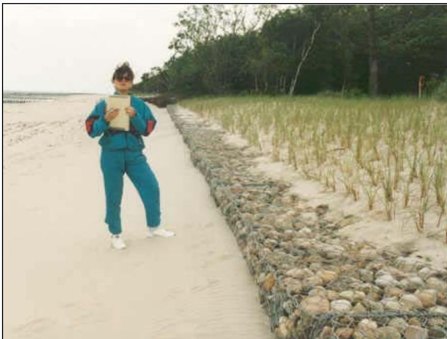
*Fig. 24: Medium seawall, slope behind the seawall revegetated, region of 8 km, 1994 (photo by K.Furmanczyk).*
