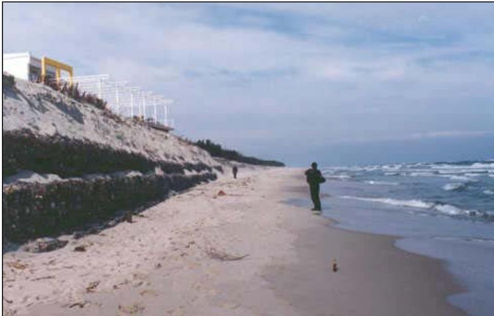
*Fig. 22: Eroded dune, opened and visible gabion seawall, Jurata, 1995 (photo by K.Furmanczyk).*
