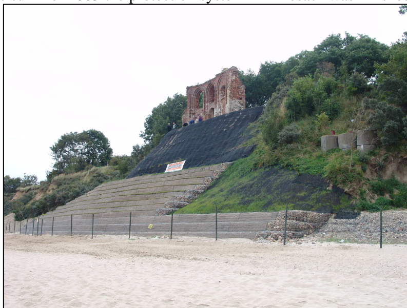
Fig. 7. Combined protection system in Trzesacz 2005. [Phot. J.Stodolny].
