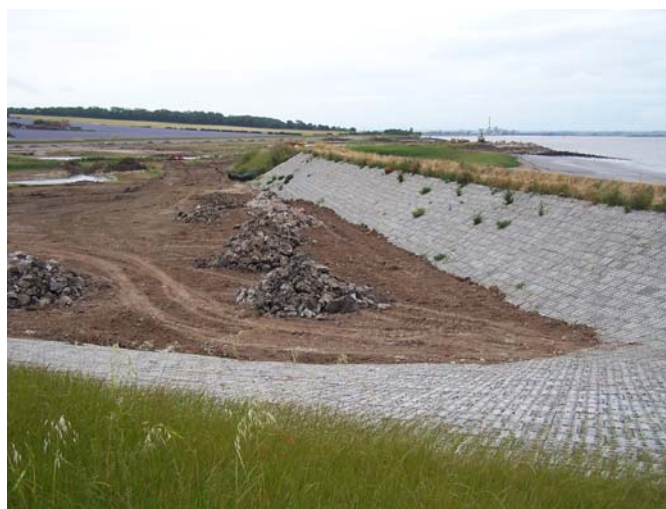
Figure 1.10: Site preparation works for Chowder Ness managed realignment site in July 2006 immediately prior to the breach (Humber Estuary, UK).
