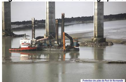
Figure 25.5 Normandie bridge piers protection
