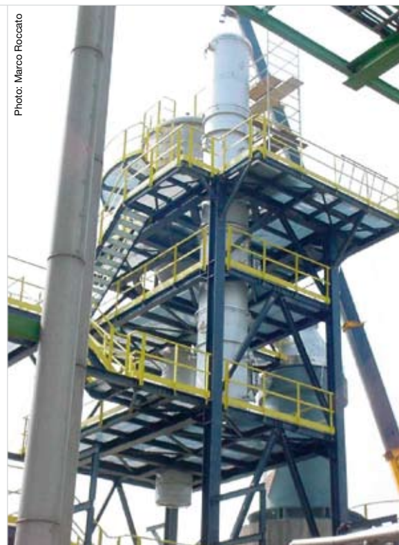
Details of the new plant showing the stripper (top) and evaporator (bottom right).
