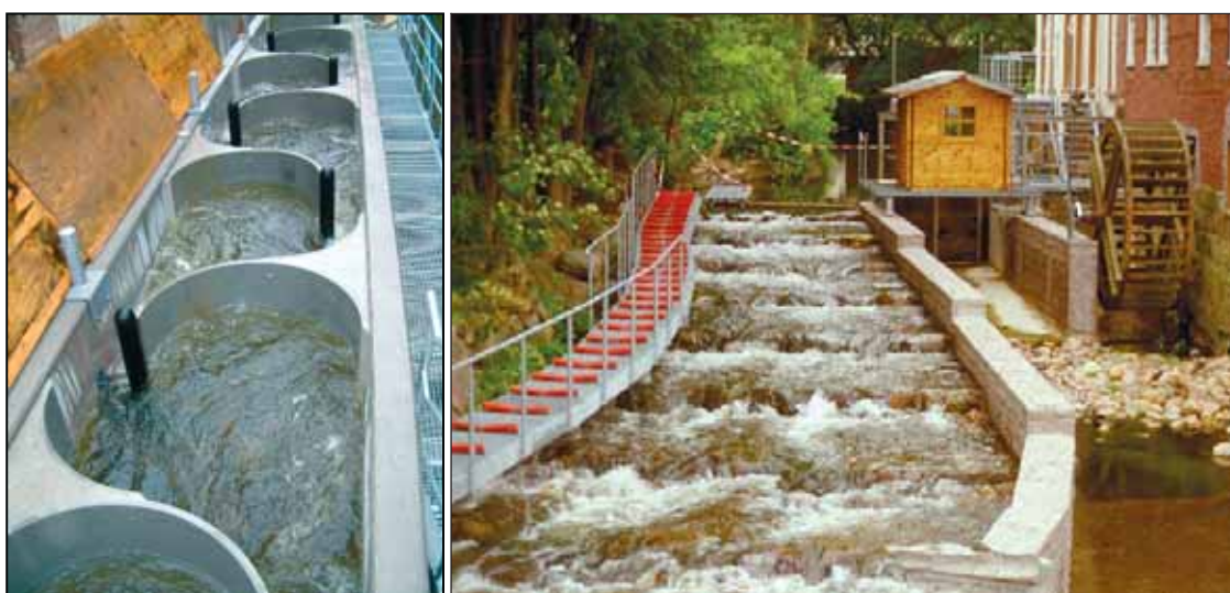
Figure 4: Helix-type Fish ladder at Power Plant Ralsdorf (left side). Fish ramp with canoe path in Malente (right side).
