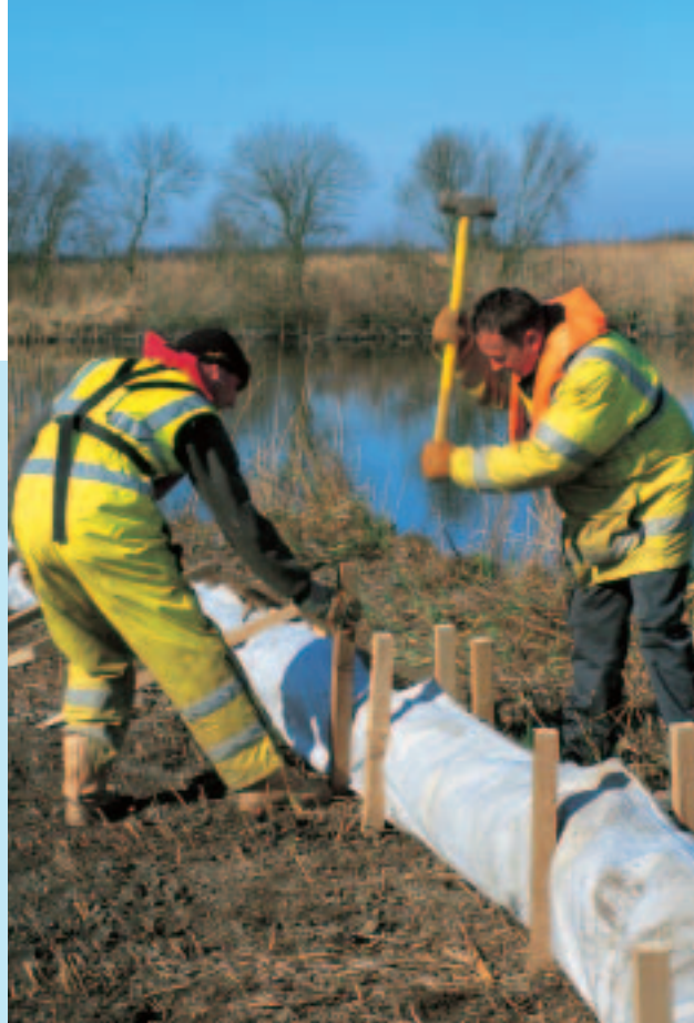
Fleet Dyke, South Walsham Broad: old dredgings are removed to form a flood bank and public footpath. Coir rolls are then secured in place to reduce boat wash when water levels are high.
