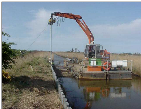
Steel piling installation, Waxham New Cut
