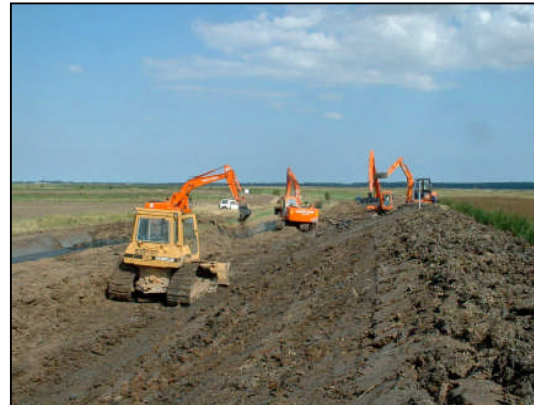
Floodbank strengthening, Reedham Marshes, River Yare
