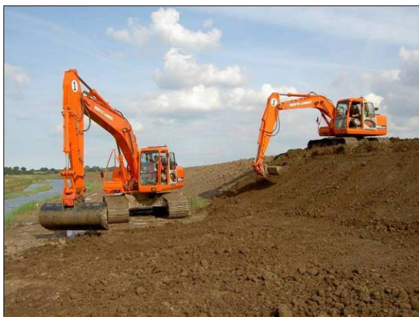
Topsoiling a strengthened bank
