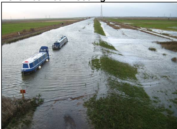
Overtopping, Haddiscoe Cut
