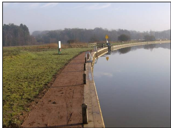
Completed mooring extension
