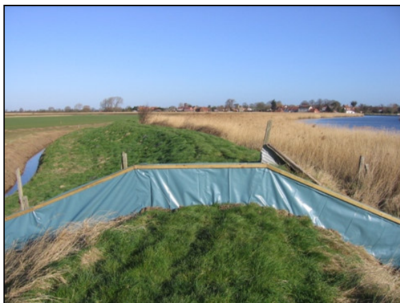
Fencing to protect a population of lizards whilst working on an adjoining length of bank
