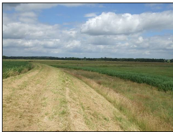
Strengthened bank at Cantley 1 year after completion
