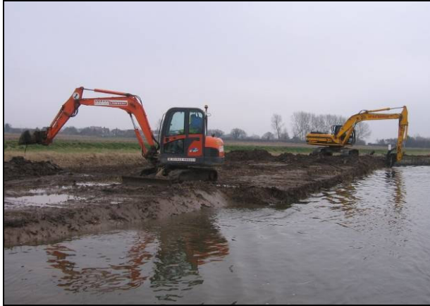
Piling removal, River Ant
