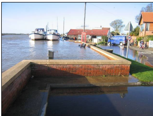
Reedham floodwall in operation, November 2007
