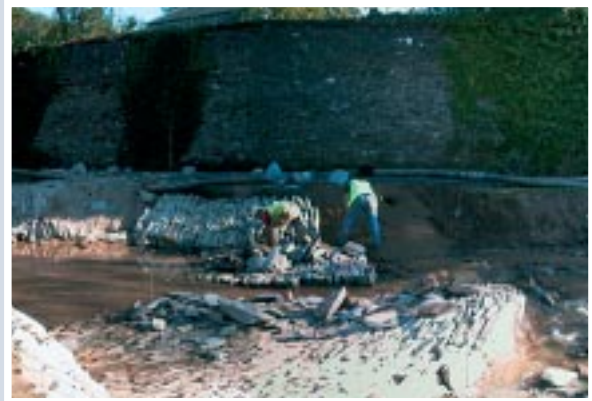
▲ Enhancing river flows - stone riffles near the village green, laid to mimic natural rock strata
