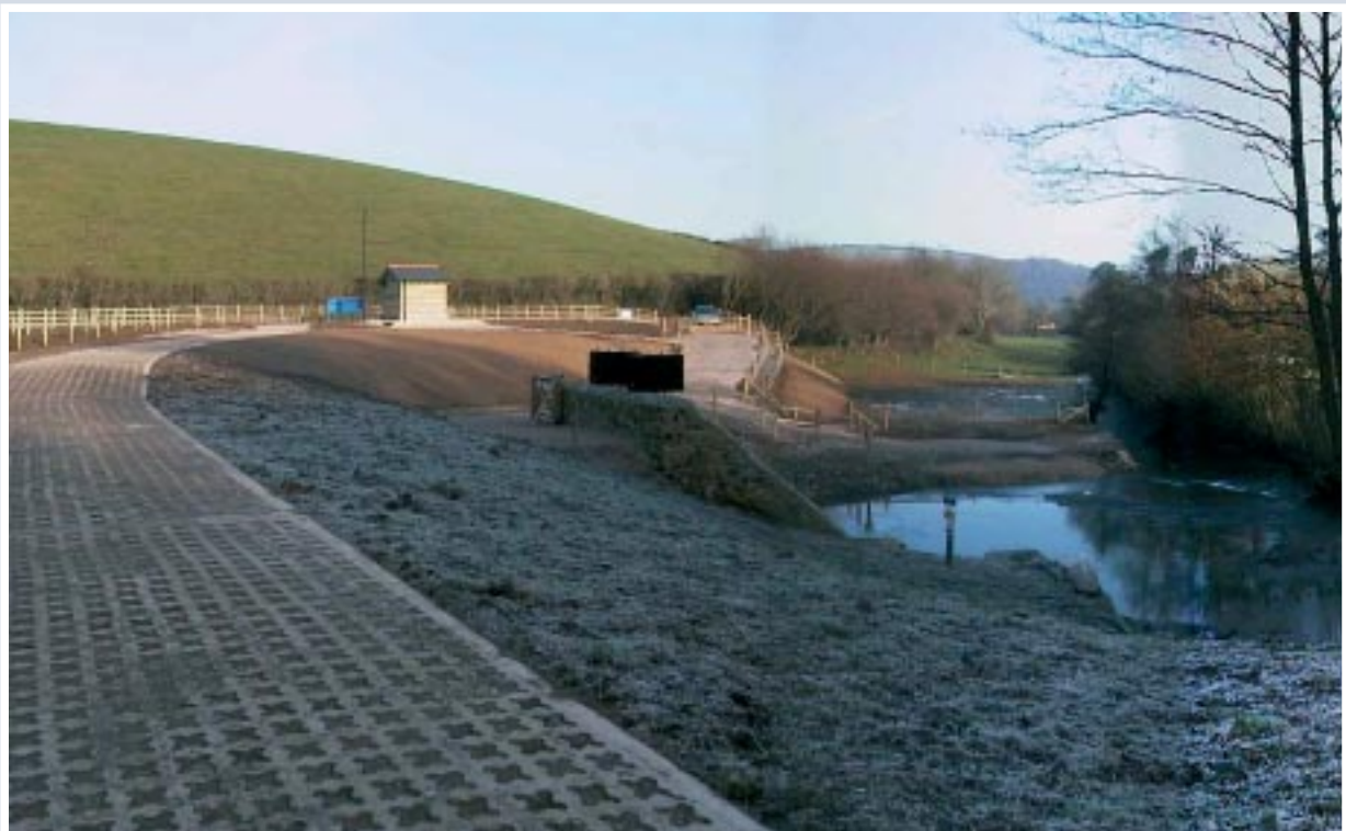
▲ The crest of the dam - nearing completion in 2002
