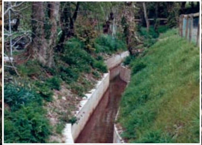
▲ The mill leat has been restored to preserve its function
