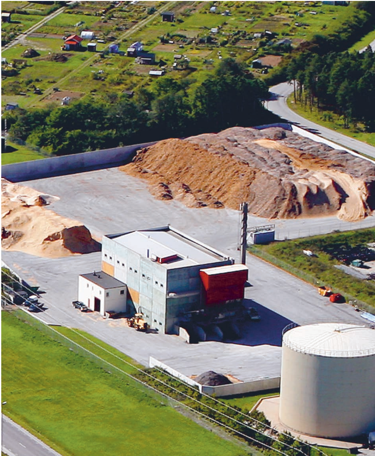
THE SKRUBB HEATING PLANT • PHOTO: GUNNAR BRITSE
