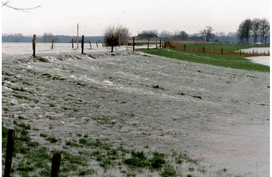
Figure 2-7 Flooding due to a dike overflow
