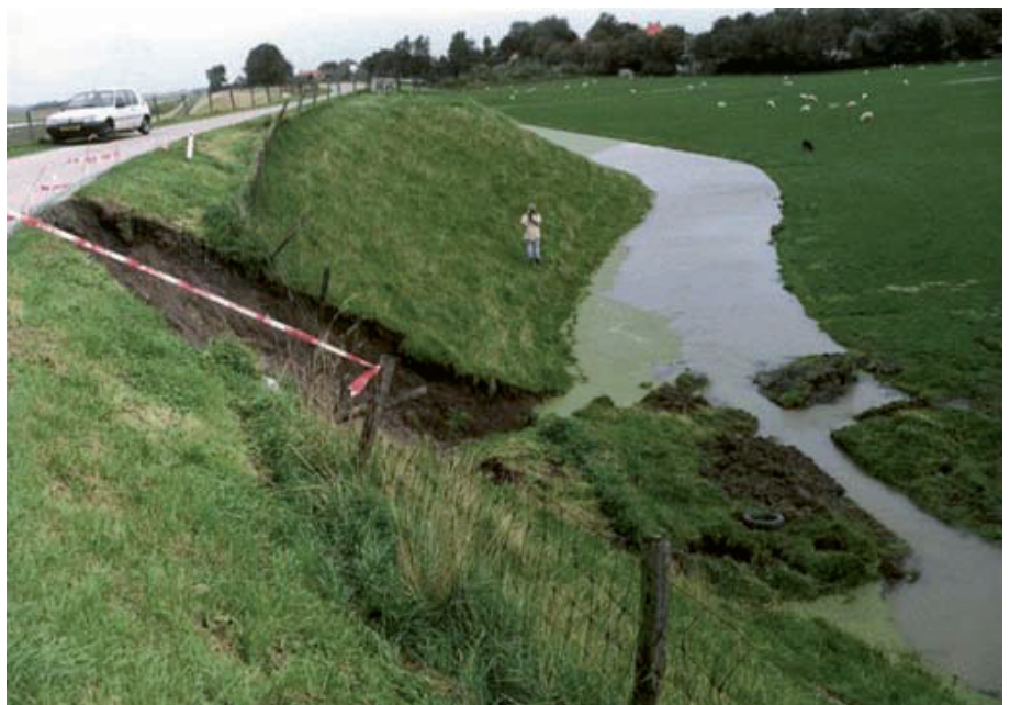
Figure 2-11 Example of sliding of the inner slope.
