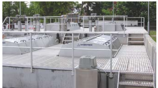
Drum and disc filters from the Copenhagen demonstration facility. The sampling unit is shown in the foreground. The water runs by gravity through both filters and the UV-station.
