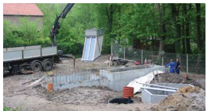
Installation of the lamella separator in the structure. The left structure is the overflow structure while the right structure is for the installation of the lamella separator.
