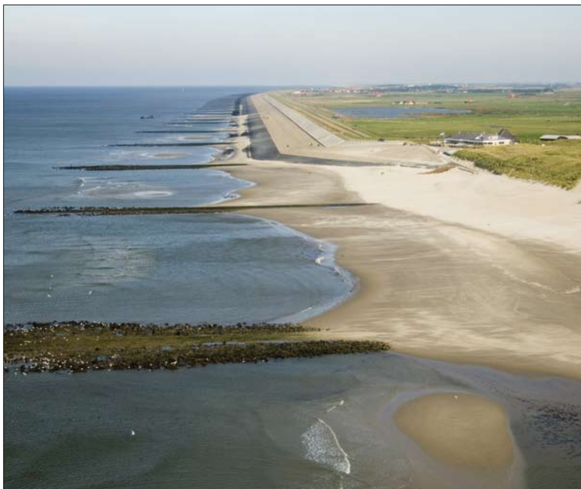
Figure 4.4: The Hondsbosse sea dike in North-Holland (NL) under influence of coastal erosion (source: RWS)
