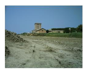
Other excavation activities regarded the canals, dug by a mechanical dredger. By and large 4000 cubic metres of sediment has been dug from the Salt works canals.
