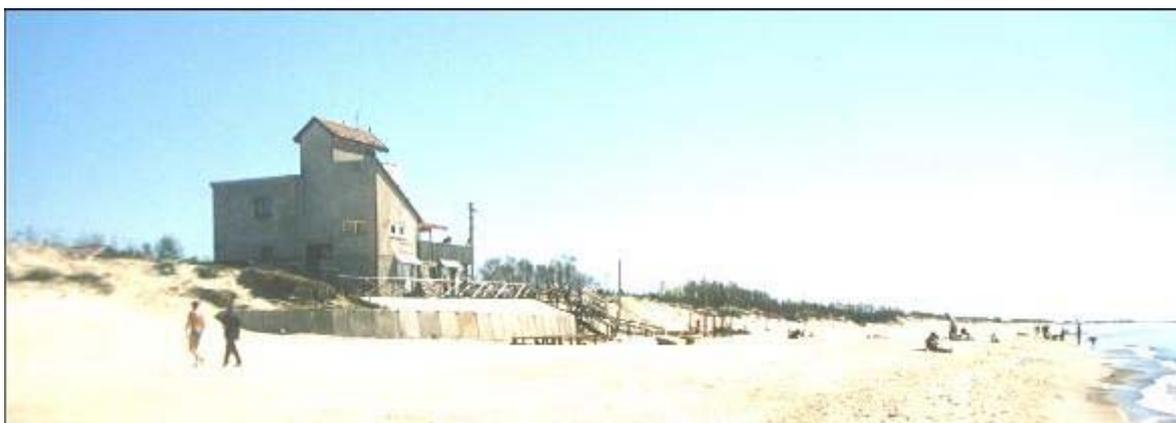
*Fig. 3: Melnrage rescue station and leisure facilities with the exposed concrete revetment on the retreating beach. Photo: E. Paplauskis, May 2001.*
