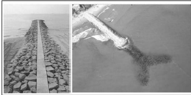
Fig. 3 – Two images of groynes realized on PONTINO littoral
