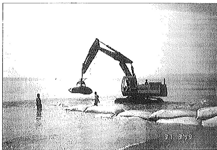
Fig. 3. Submerged groin construction
